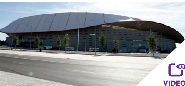
Construction of the cover of Wanda Metropolitano
